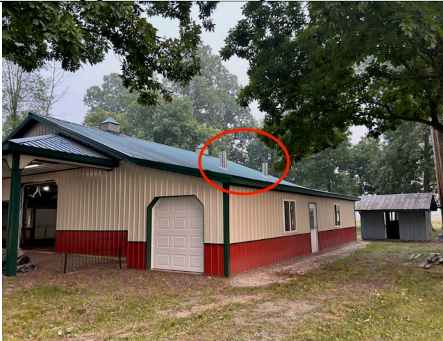
Our Rainsville shop showing 2 of the 3 new chimneys on the west side.
