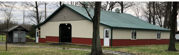
Our building gets new metal siding. Overhead doors should be installed shortly.
