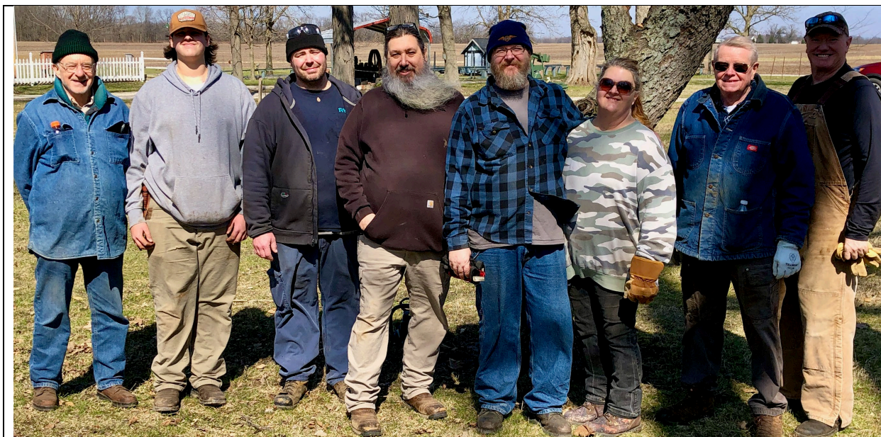
Rocky Forge crew on March 26 helps prepare the Rainsville Shop for major renovations including metal walls and doors, electrical work and forge ventilation systems.
