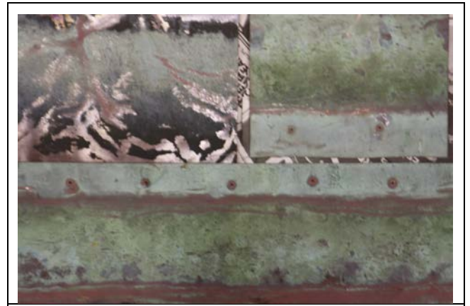
Natural patina on three pieces of copper gutter.
