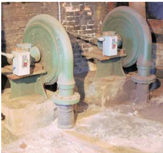
Pair of forge blowers, American Blower Corp. All of the shop's forges, both gas and coal-fired, are supplied with forced air from blowers like these.
