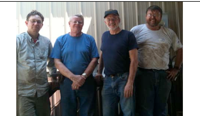
After a hard morning removing the line shaft, KJ, Ted, Dominick and John are tired and a little grimy.
